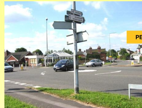
These smaller versions of regular traffic circles are designed for narrower residential streets. The center island is usually painted and slightly domed. Larger vehicles can drive over the edges of it. Where space permits, small islands on each approach deflect traffic away from a straight path. All entering traffic yields to the left. Traffic circles reduce travel speeds.
