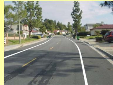
Striped parking lanes added to the roadway top reduce the effective width of the traveled way. This helps to reduce traffic speeds.
