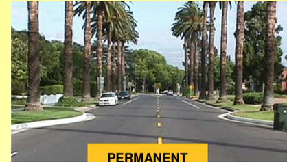
Mid-block chokers are curb extensions located between intersections. They can leave the cross section with two narrow lanes.
